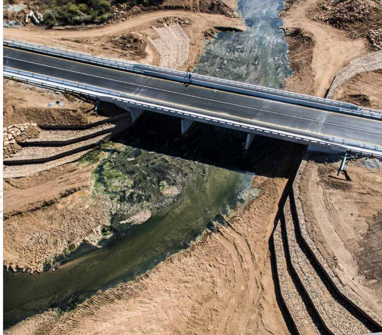
Construction of the Tolwane River Bridge – Mabopane Gauteng
