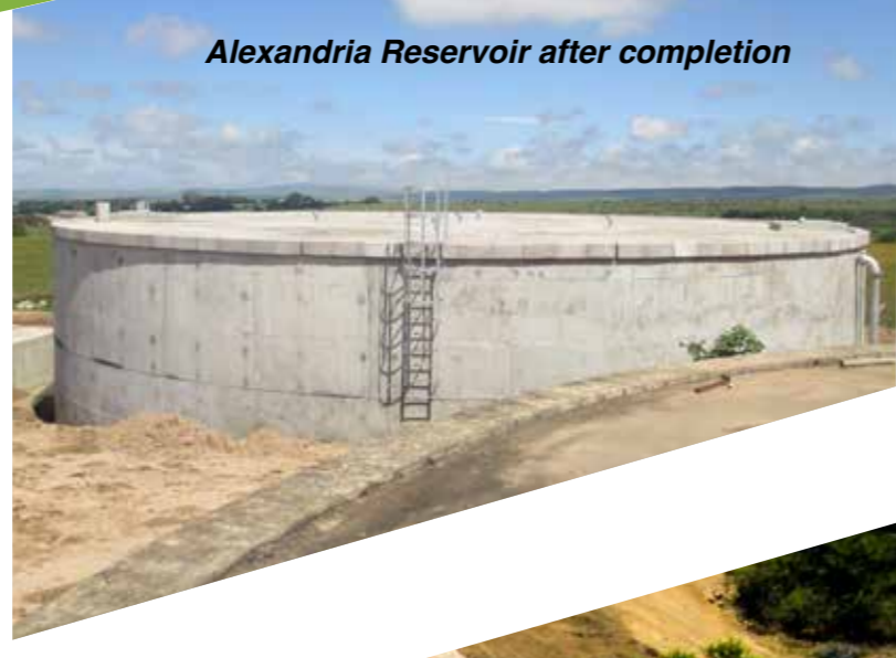
Reservoir under construction at Alexandria
